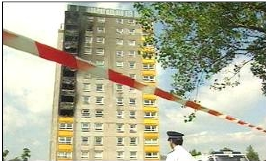
Figure 2: Apartment building fire, Irvine, Scotland (source: BBC Online Network, 1999)
