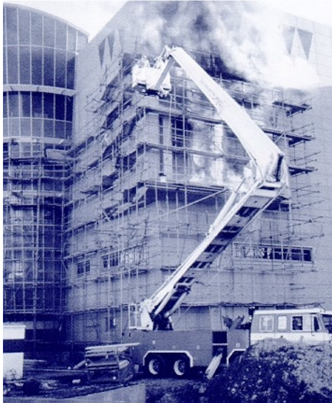
Figure 4: Museum construction fire, Wellington (source: NZFS, 1997)
