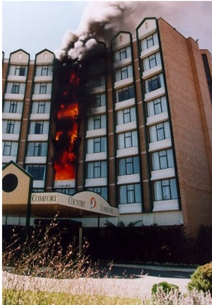
Figure 3: Motel fire, NSW, Australia (source: NSWFB, 1999)
