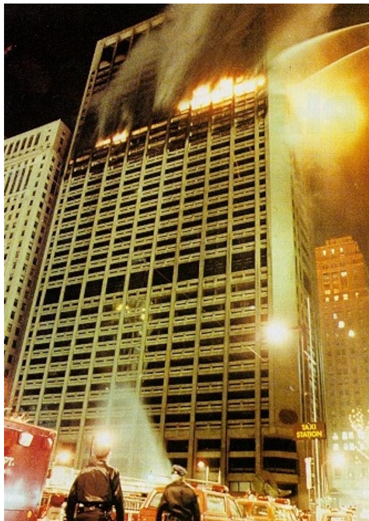
Figure 6: One Meridian Plaza fire (source: Klem, 1991)
